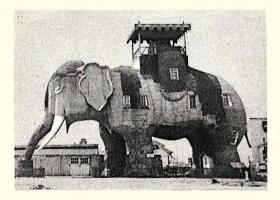
This elephant-shaped house at Margate City, N. J., has 22 win dows. It consists of over a million pieces of wood, 8560 ribs, 200 kegs of nails, 12,000 square feet of tin, four tons of bolts.
