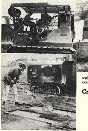
Top-Equipped with a 100-horsepower Diesel engine, this machine tamps down new asphalt and concrete roads with a tamping pressure of 60,000 pounds. Bottom-This hand operated tamper exerts 600 pounds pressure.
